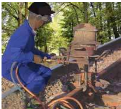
Figure 3.11 Thermit process for joining railway tracks
