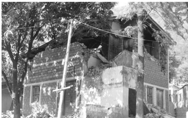
Figure 7.1 : A Damaged Building Due to an Earthquake
