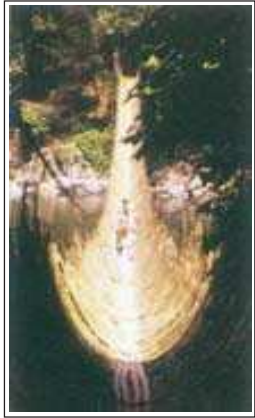
Figure 6.7 : Rope Bridge (Arunachal Pradesh)
