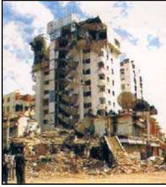
Fig. 3.3a: Destruction caused by an Earthquake at Bhuj
