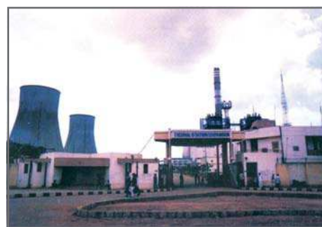
Fig 3.12: A view of a Thermal Power Station
